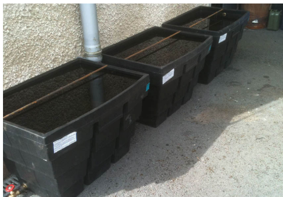
Figure 2. Bioboxes outside of Sligo drinking water treatment plant (photograph by Sara Meehan).
